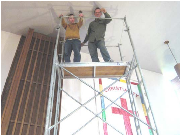
Lighting repair - October 5, 2009
