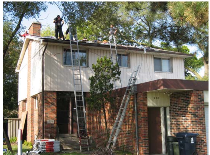
Rectory re-roofing - October 10, 2009
